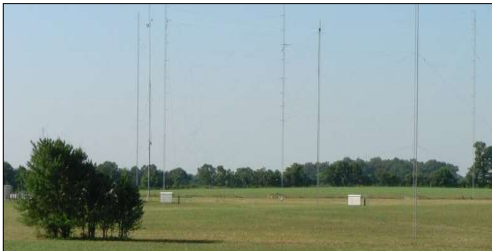
WWRB antenna complex
