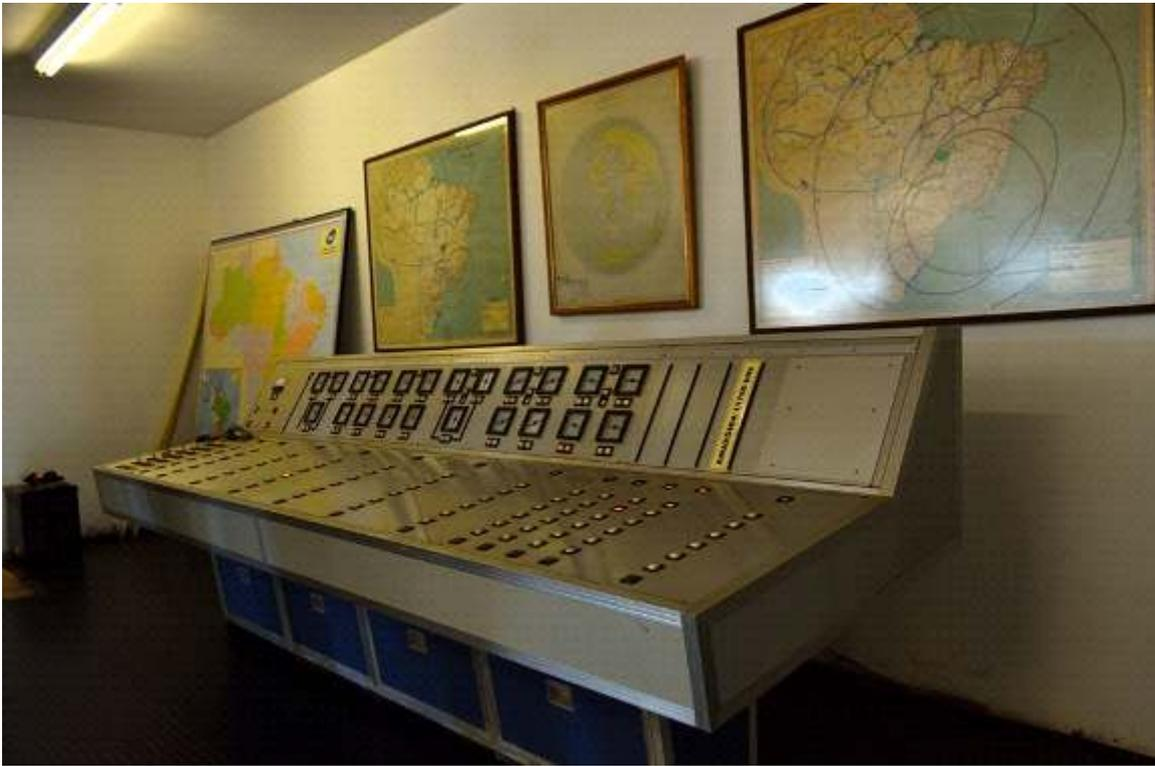
By this console (above) we can see different maps with the radiating lobes of the antennas, and the theoretical coverage of transmissions from different areas of Brazil and the world.
